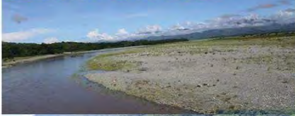
Aggrading river due to increased elevation of riverbed
