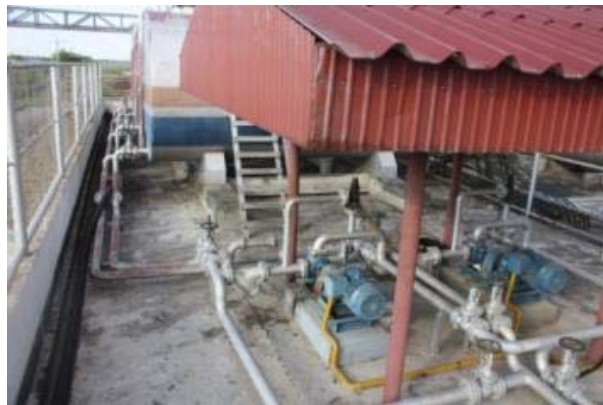
Drips & spills at fill-points (external to bunded tanks) can only drain to stream
