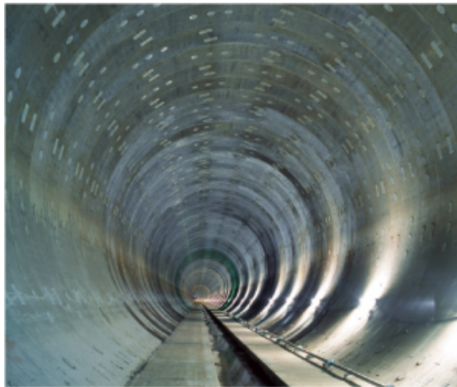
The Wada-Yaoi trunk sewer
