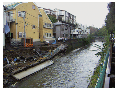
Damage to river bank and overflow to inland In Nakano-Ward
