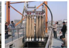
Checking Membrane Condition
