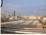
Hainan project (10.800m 3 /day)
